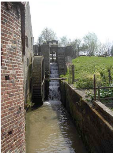
Figure 2: The watermill (left) used in Belgium converts the translational energy of the flowing water into mechanical energy that can be used to run various processes, through the mechanism seen in the right picture.
